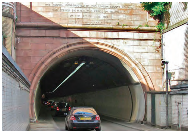
Southern portal of the Rotherhithe Tunnel taken from the pavement which runs all the way through. Note the inscription above the arch: This tunnel constructed by the London County Council was opened by H.R.H The Prince of Wales K.G. on the 12th June 1908. Maurice Fitzmorris C.M.G. Engineer
